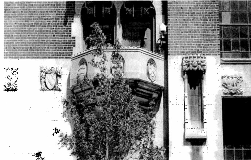
The Calumet Plant is finely detailed with a variety of Gothic-style ornament in metal, terra cotta, and stone. Top: Window spandrels are detailed with Gothic-style foliate metal ornament and terra-cotta shields bearing symbols historically associated with the printing trade. Above: Carved stone ornament, including historic printers-marks and foliate-detailed Gothic niches, are clustered at the building's first floor. Right: A detail of one of the carved-stone printers-marks.
